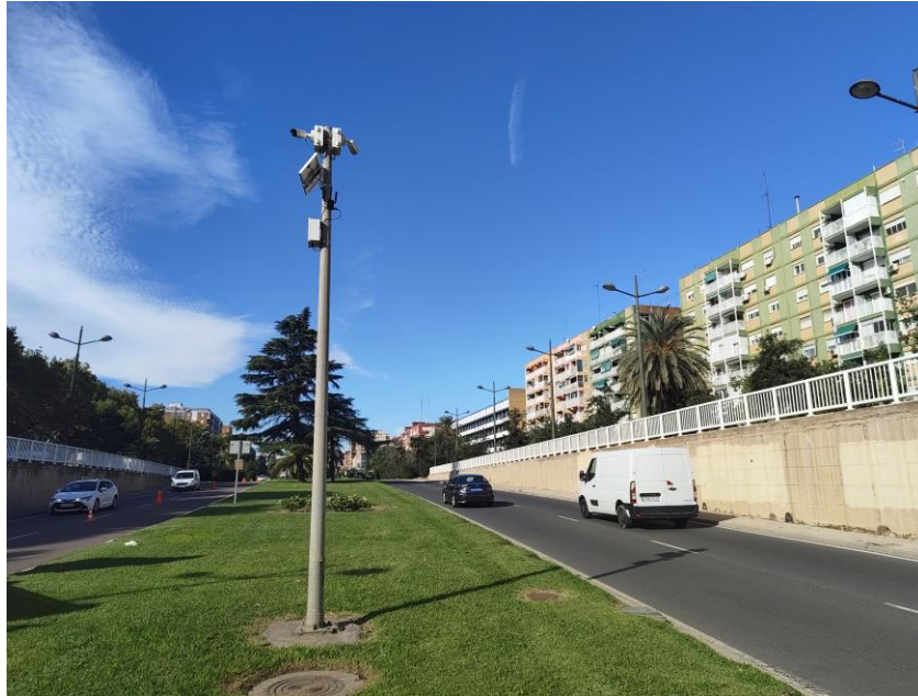
Figure 11: Installation of radarMovAvCid.
