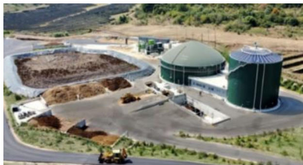
Figure 8.6 Aerial view of the biogas plant in Preveza, Greece
